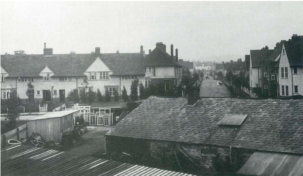
Fig. 35 View of newly built housing across the on-site builder's yard in 1909 http://www.hgstrust.org/history/images/photograph_4.jpg
