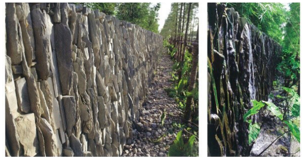
Fig. 47_ Cascade aerates and cleanses river water
