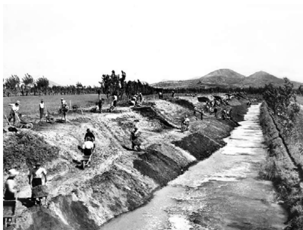
Fig. 16_ A vast project of ditch digging
